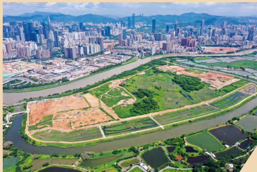
Hong Kong-Shenzhen Innovation and Technology Park (under construction)
