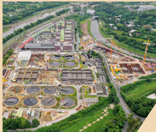
Shek Wu Hui Sewage Treatment Works
