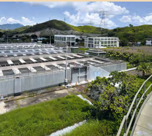
Sheung Shui Water Treatment Works
