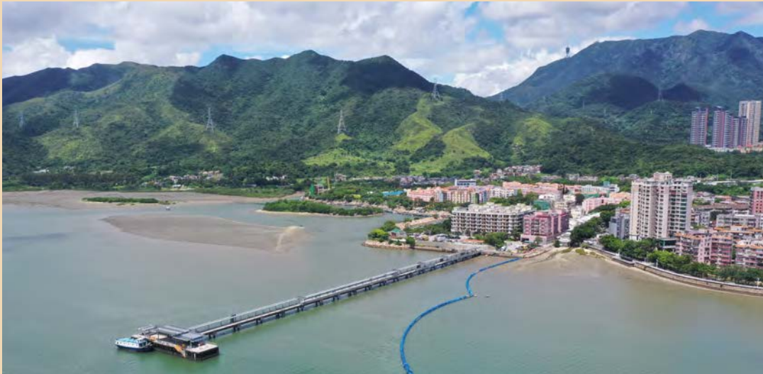
Sha Tau Kok Pier
