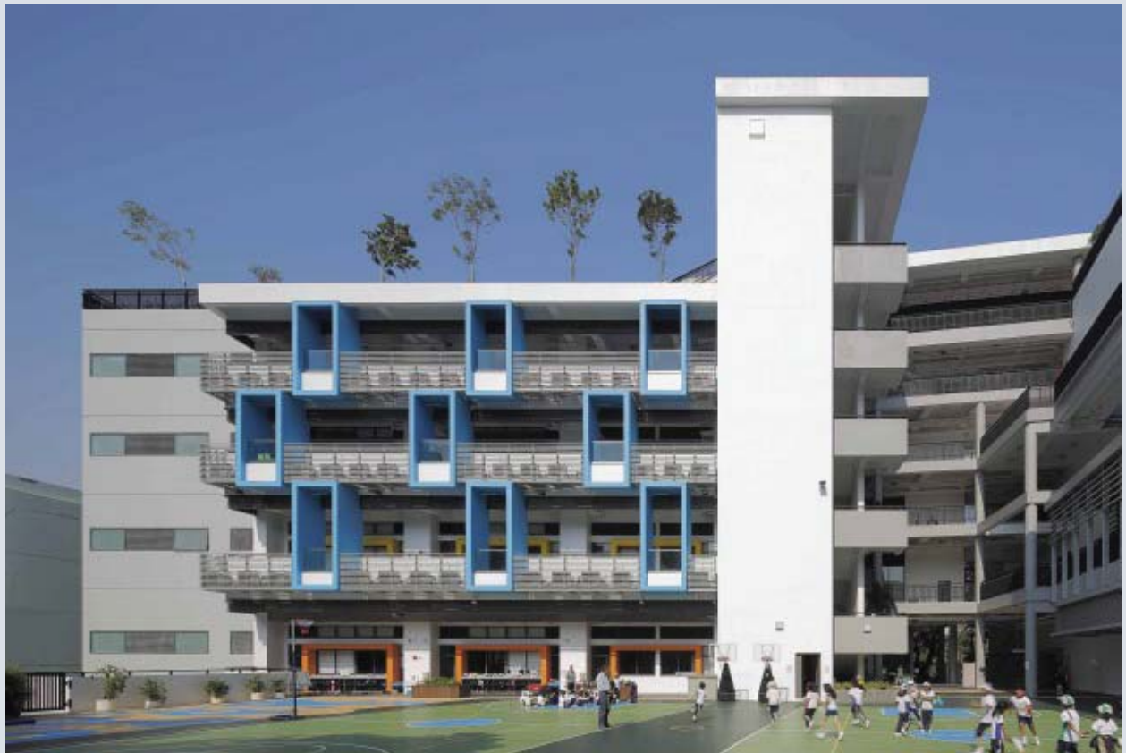
Redevelopment of Kowloon Junior School, BEAM Plus (New Buildings) Certification
