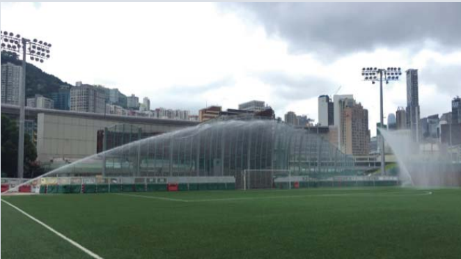
Water harvesting for irrigation at sport pitches at Happy Valley Recreation Ground
