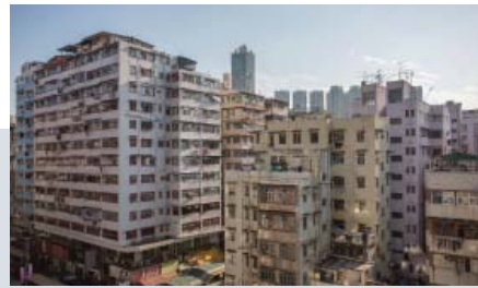
Existing building stock in need of maintenance and repair
