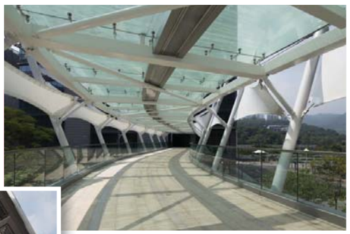
Footbridge with fritted glass tops & sun shading tensile - minimise solar heat gain and insulate western sun
