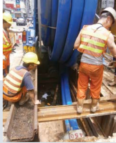
Performing mains rehabilitation work in Tolo Highway
