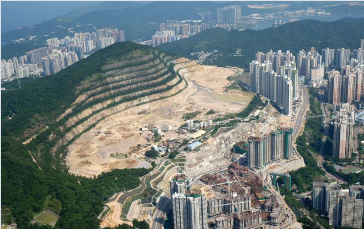
Anderson Road Quarry Development site has potential for PV installations
