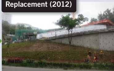
Replacement and replanting works carried out on site
