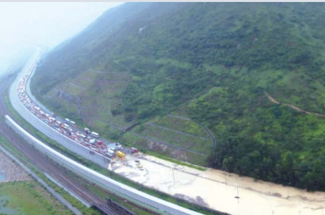
North Lantau Expressway paralysed by debris flow during June 2008 rainstorm
