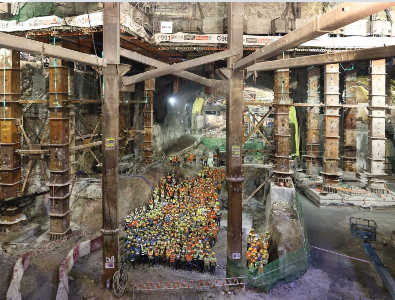
Extension of Admiralty Station involve many engineering challenges
