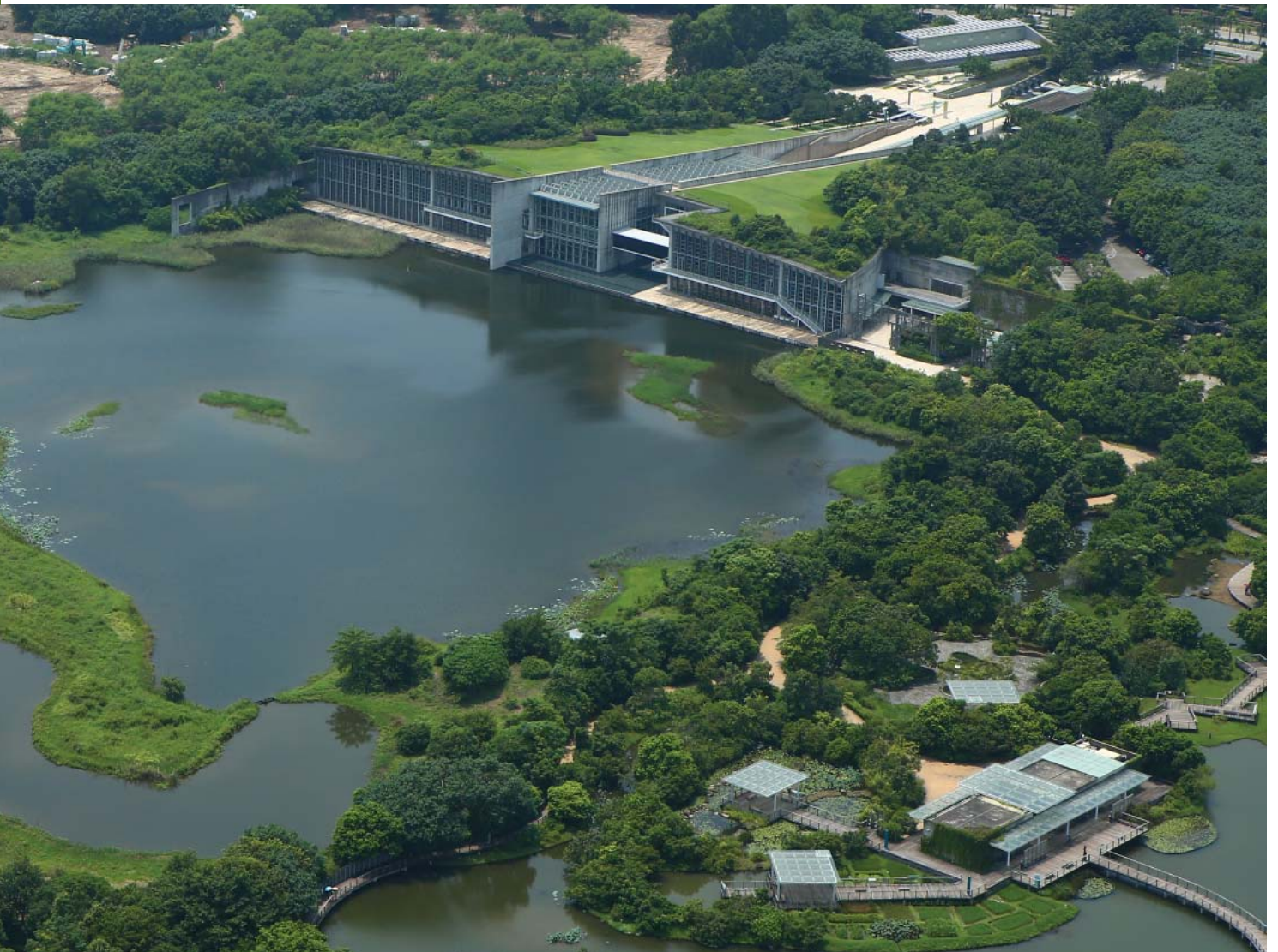
Green roof of Hong Kong Wetland Park, Tin Shui Wai
