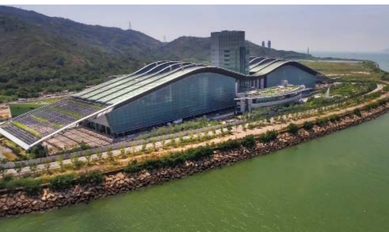
T • PARK Sewage Treatment Works
